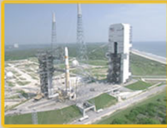
Fully Activated CCAFS Launch Facilities
